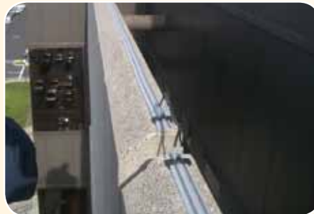
Bird Barrier's Quick-Connectors are used to bridge a 6-inch gap in these concrete decorative features.
